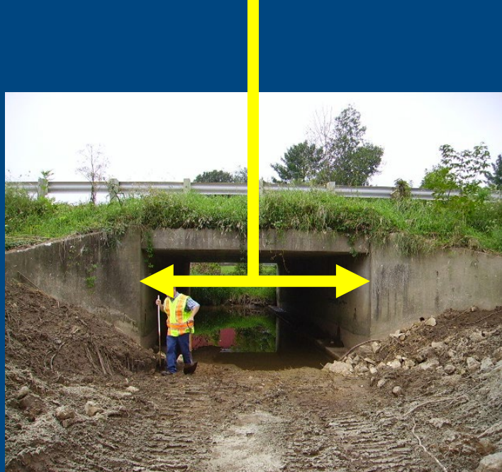
Buried Concrete Rigid Frame (no floor)
