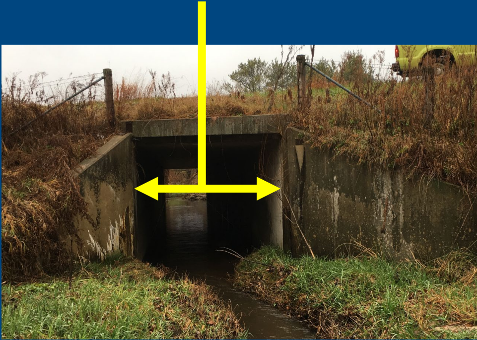
Single-Cell Concrete Box Culvert
