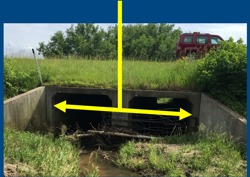
Multi-Cell Concrete Box Culvert
