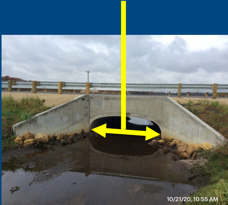
Precast Concrete Arch
